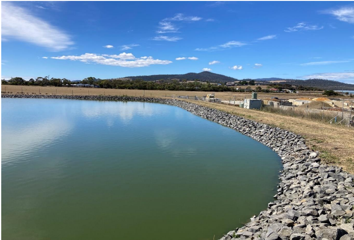
Figure 7 Erosion Protection Dunalley Lagoon No.3
