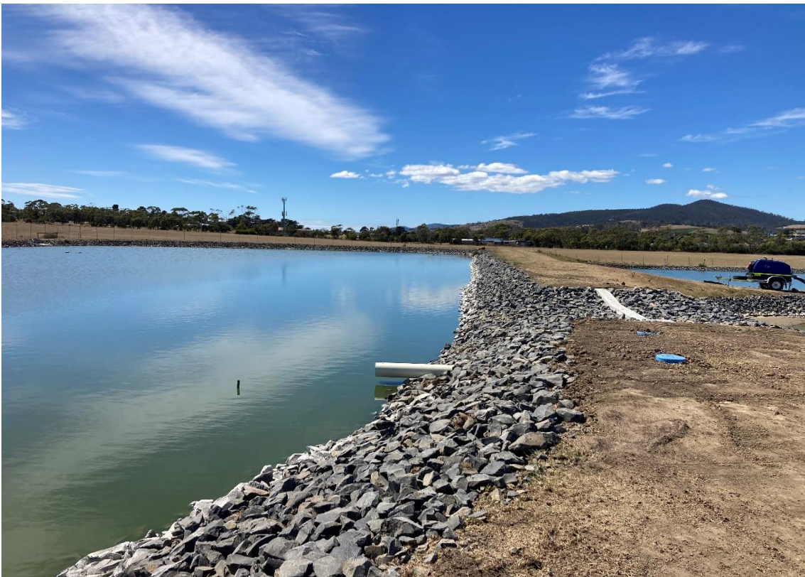
Figure 6 New outlet pipe, and emergency spillway Dunalley STP.
