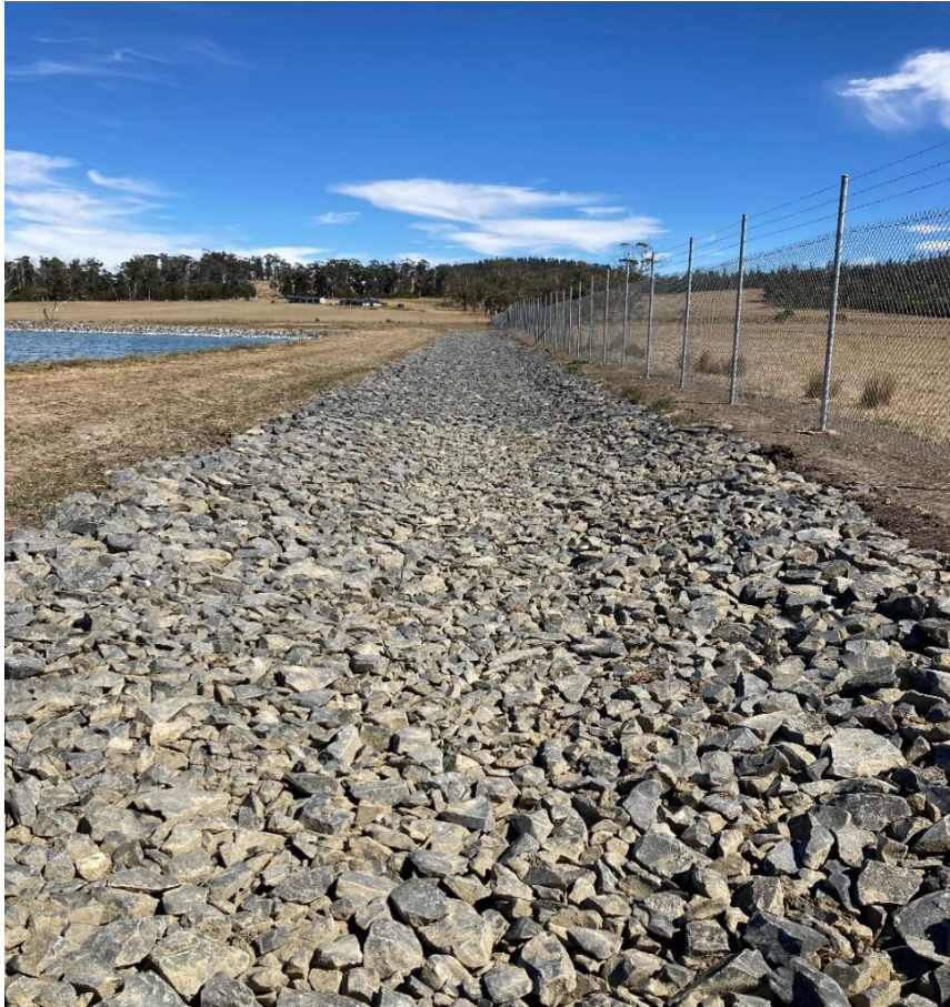
Figure 8 Stormwater Cut-off drain Dunalley
