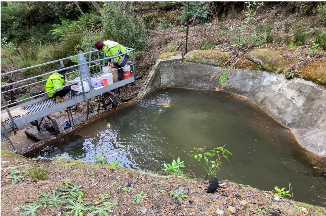
Figure 11 Mole Creek Weir Repairs
