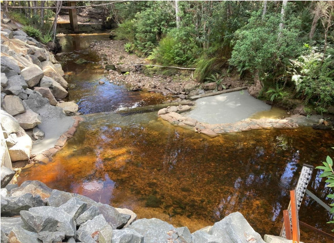
Figure 10 Manuka River Weir Repairs
