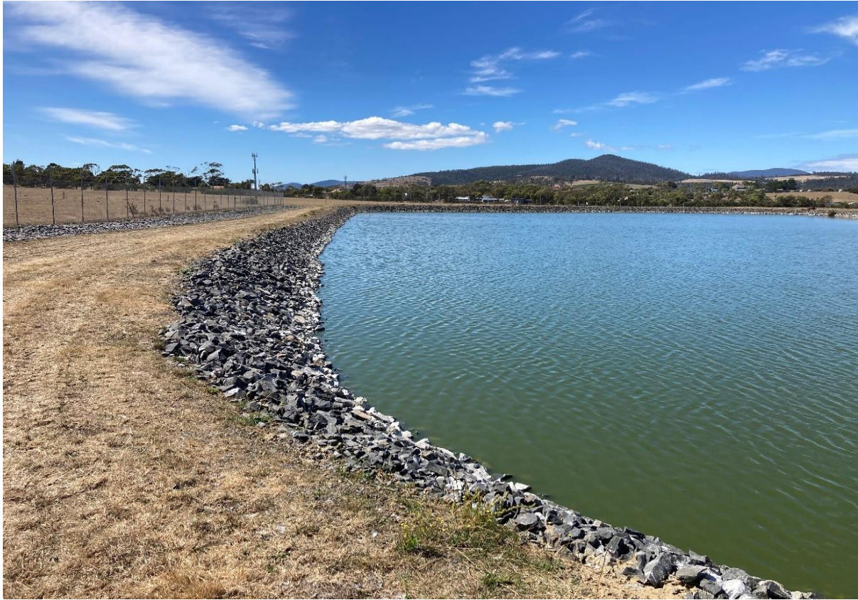
Figure 9 Erosion Protection Dunalley Lagoon No.1
