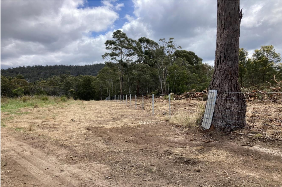
Figure 5 Bradys Creek Dam Boundary Clearing and Fence Installation
